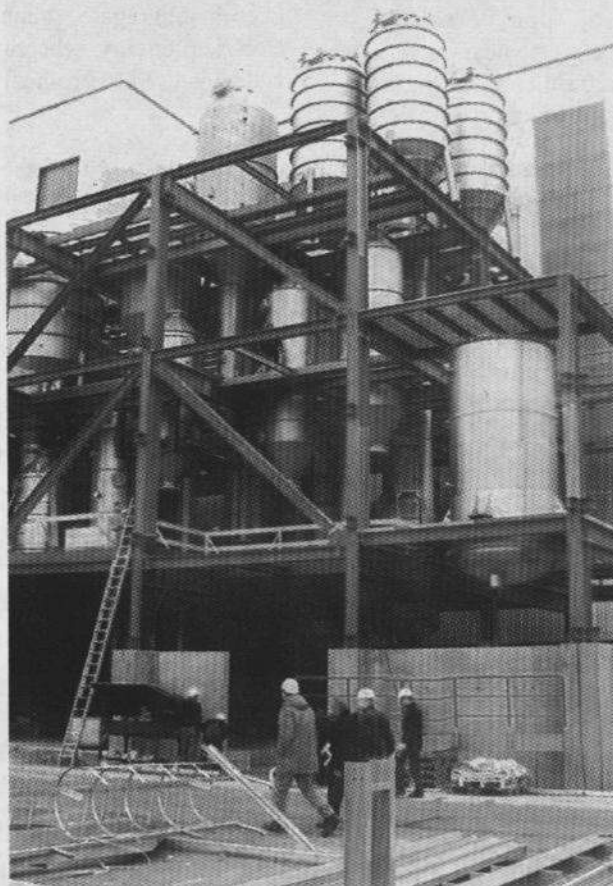
Fig. 5. New 7-effect recrystallization plant at Bad Friedrichshall, under erection
